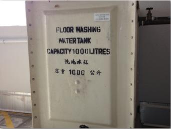
Rain Water and Air Conditioning Condensate Water Harvesting System (left: reclaimed water pump room, right: floor washing water tank)
