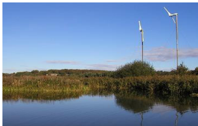
Figure 1. The two 25kW 2-bladed wind turbines. Note the man-made lake in the foreground.
