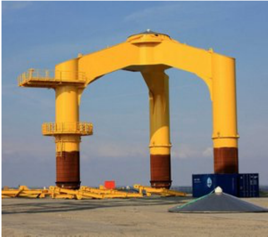
Figure 2.12 - BARD first tripile foundation [37]
