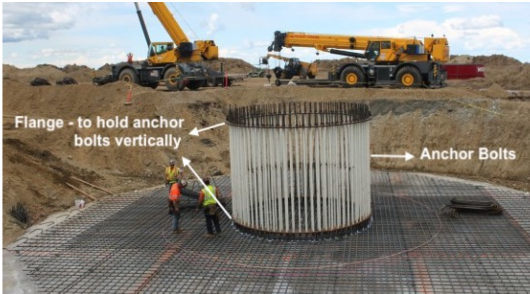
Figure 2.4 - Concrete foundation with anchoring bolts & flange [24]
