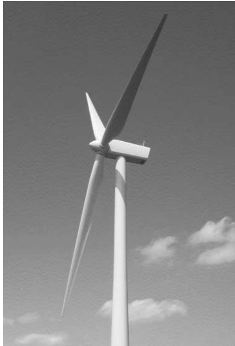
Figure 1. A typical modern wind turbine.
